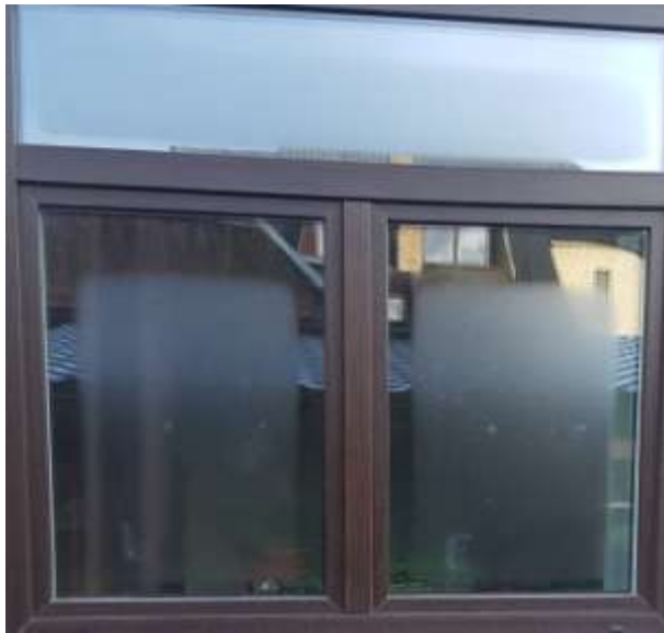
Example: Condensation forming on the glass surface
