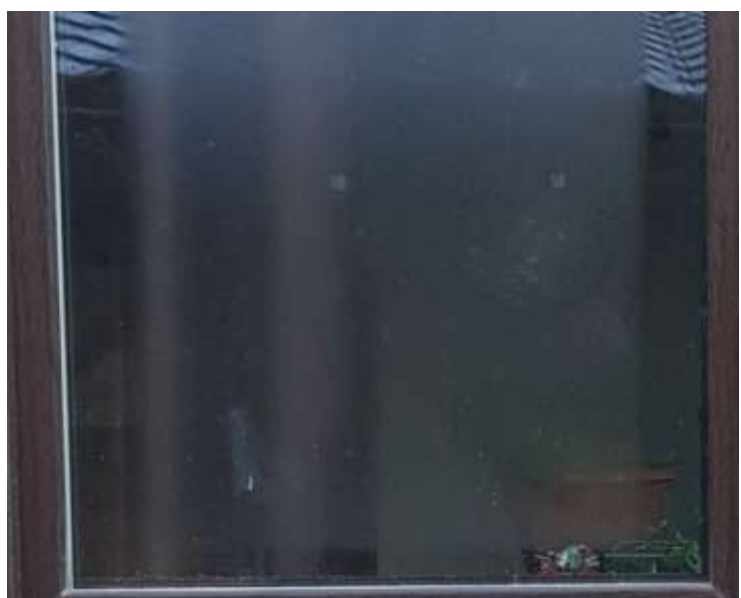
Example: Marks on the glass surface from vacuum lifters or gaskets
