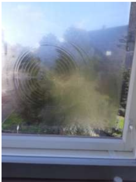
Example: Marks on the glass surface from vacuum lifters or gaskets
